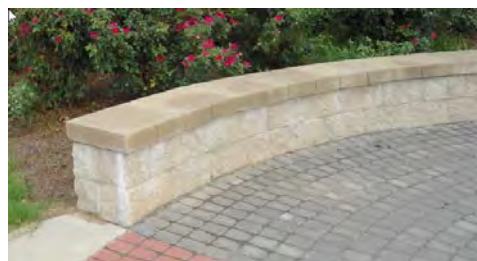
Split-face CMU retaining Wall with cap
