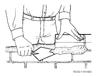
i. Cut off any excess mortar.
