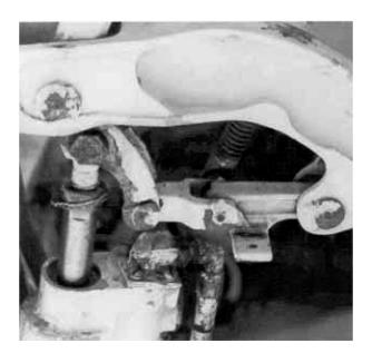
Figure 3-19. Steel Corrosion Products (Rust)
