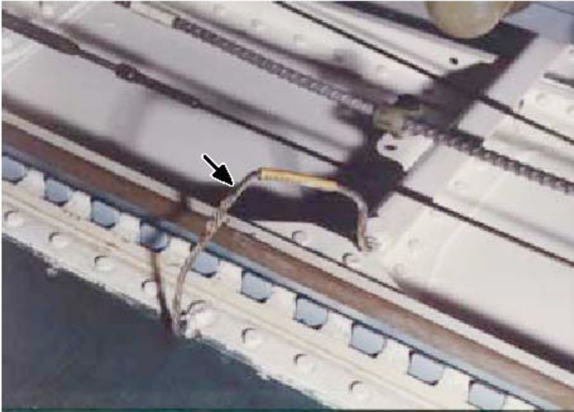
Figure 7-4. Bonding Cable from Airframe to Graphite/Epoxy Avionics Bay Door
