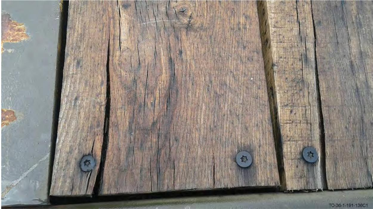
1.6.3.4 Scratches and Marks. Scratches, tool marks, compression and/or stress marks which do not impair structural integrity or components are ordinarily of no significance and do not render an item unacceptable.
