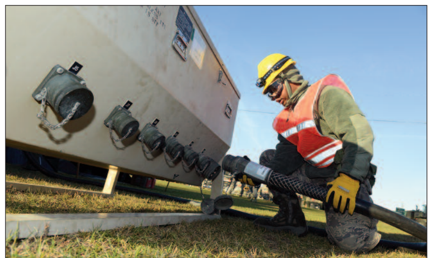
Senior Airman Vacarro Robinson, 51st Combat Communications Squadron power production technician, connects generators which power the unit's communications equipment during a mission simulation exercise Dec. 6 at a Georgia Air National Guard Combat Readiness Training Center in Savannah.
