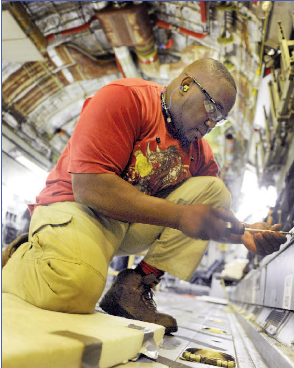
Derrick Chatmon, 562nd Aircraft Maintenance Squadron aircraft mechanic, installs kick panels on the C-17 being modified with an on board fire suppression system. The system operates much like a controlled fire extinguisher, dispersing inert gas which prevents an aircraft from being engulfed in flames when it's hit during enemy engagement.
