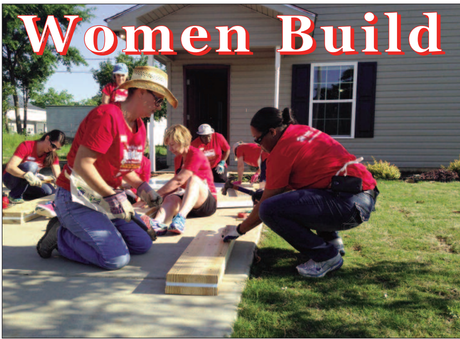
Courtesy photo by ASHLEY WILLIAMSON Senior Master Sgt. Sally Perez (left) and Master Sgt. LeSharee Hicks (right) from the 78th Medical Group make sure the header is properly aligned before nailing it together. The header will help support the windows and doors on Nannetta Tennyson's home – the 50th Habitat home in Houston County. Women Build volunteers built headers and jacks for Houston County Habitat for Humanity's 50th home. This was HoCo Habitat's second annual Women Build in support of National Women Build Week.
