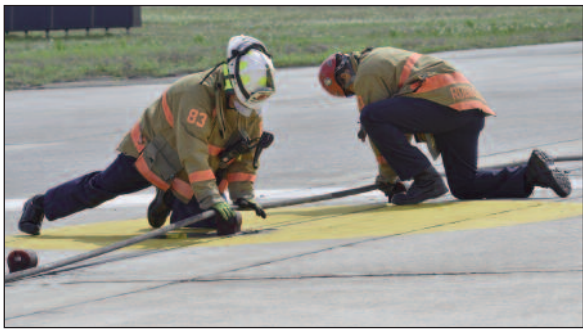
U.S. Air Force photos by ED ASPERA Base firefighters prepare the cable system prior to the F-15 landing at Robins. The use of the system was for a scheduled annual certification engagement April 8.
