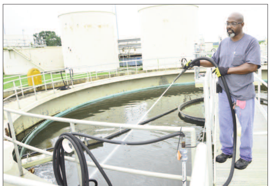
Darryl Hall, wastewater treatment operator, removes algae and other biological growth from a secondary clarifier which separates sludge from wastewater where it's further processed for discharge into the Ocmulgee River.
