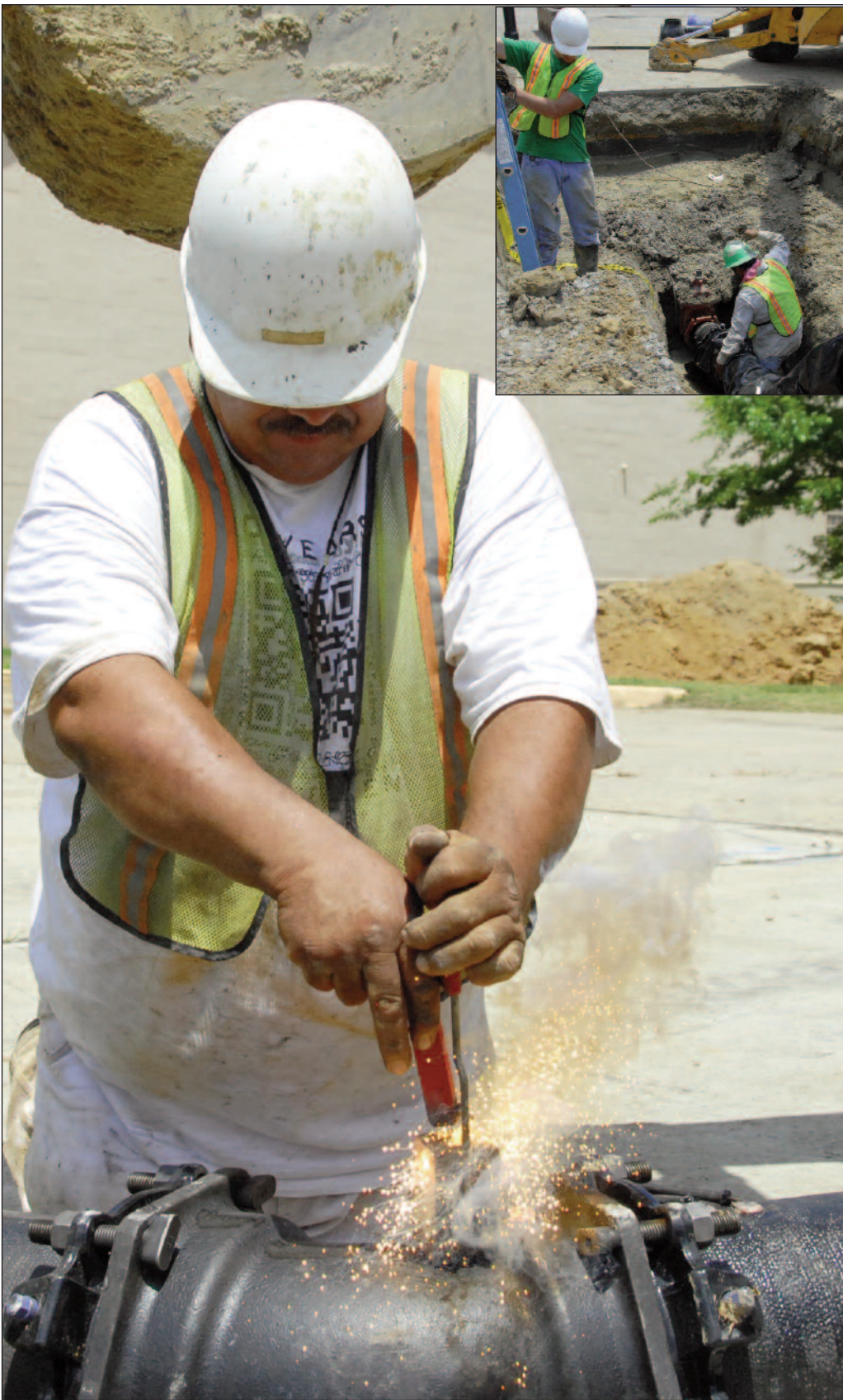
U.S. Air Force photos by MISUZU ALLEN Above, Jose Hernandez welds electrical cables to a new main waterline pipe by the base History Office. The water that goes through this pipeline is used for the building's fire protection sprinkler system. Inset Manny Nunez (right) and Tyler Belt, contractors, get down and dirty to install the pipe.
