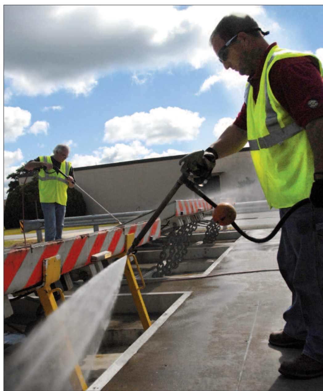
U.S. Air Force photos by MISUZU ALLEN Jon Mason (right) and Mike Middleton, 78th Civil Engineer Wastewater Plant Operator, use a pressure washer Tuesday to clean beneath the vehicle barrier at the Russell Parkway Gate. The maintenance of the barriers is scheduled to take place monthly at the Russell Parkway, Watson Boulevard and Green Street gates.
