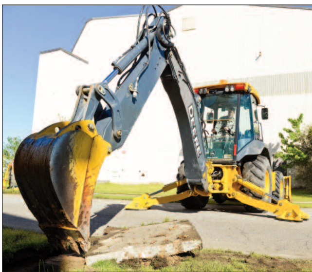
Senior Airman Shane Kilgore, a heavy equipment operator with the 116th Civil Engineer Squadron, uses a backhoe to break up and remove concrete while correcting a storm water drainage problem.
