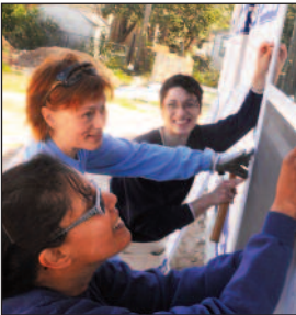
Front to back, Lt. Col. Libby Melendez and Lt. Col. Dee Ketterer, AFRC, and Michelle Hopkins, 402nd Electronics Maintenance Group, put a window in place March 16 on a Habitat for Humanity house.
