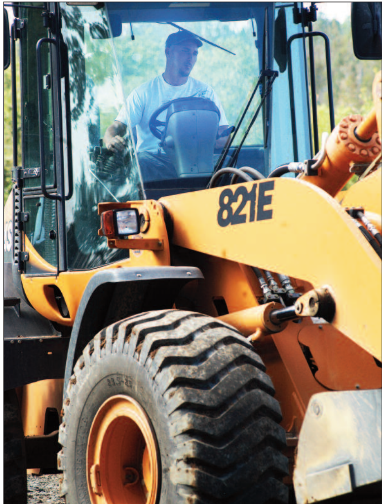
U.S. Air Force photo by SUE SAPP Matt Allen uses a loader to remove asphalt along Hannah Road Sept. 7. Hannah Road is currently closed for a major construction project to replace a damaged drainage culvert and repair the bridge.
