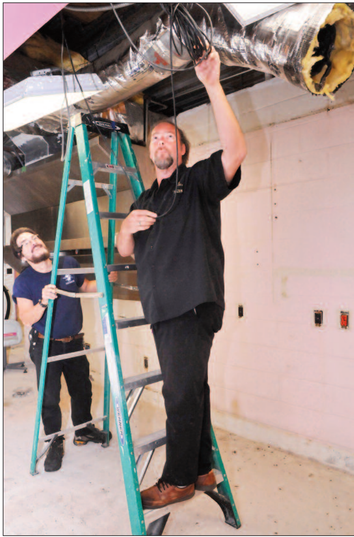
U.S. Air Force photo by SUE SAPP L-R, Fred Babcock, Robins Bowling Center janitorial technician, holds a ladder for Rick Catlett, maintenance manager, to check on some cable during renovations of the On Spot Cafe.
