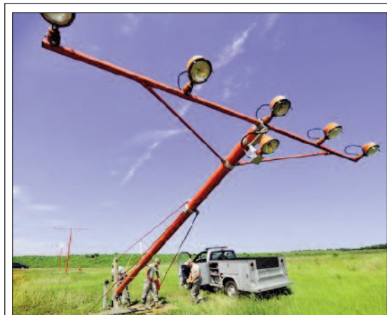
U.S. Air Force photo by SENIOR AIRMAN KENNY HOLSTON From left, Staff Sgt. Julius Givens, Airman 1st Class Justin Fleming and Tech. Sgt. Daniel Harrington repair airfield approach lighting at Shaw Air Force Base, S.C. The 20th Civil Engineer Squadron Airmen worked together to recently repair several airfield lighting lamps and re-sync flashing approach lights.
