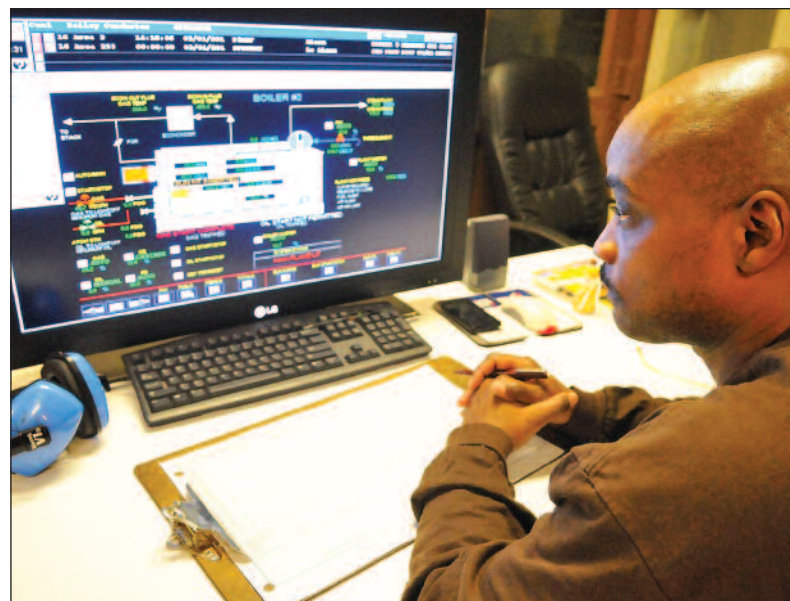
Ernest Moss, boiler plant operator, monitors boiler and steam output.
