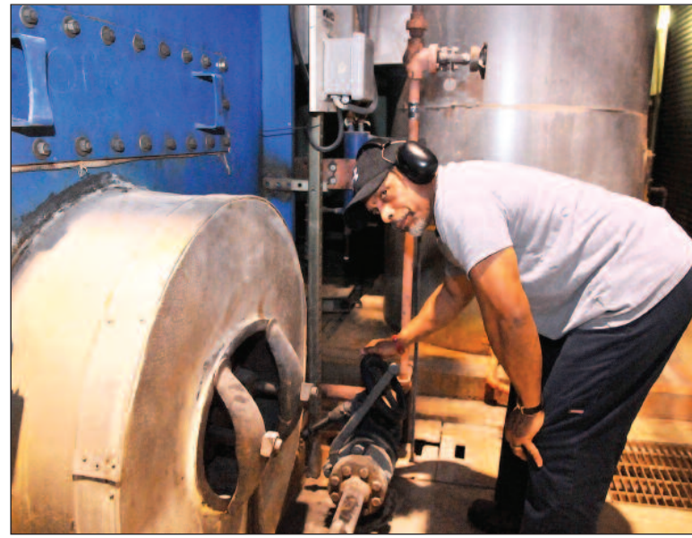
Sid Brown, 78th Civil Engineer Group Boiler Plant operator, works to remove sediment from the water in a boiler.
