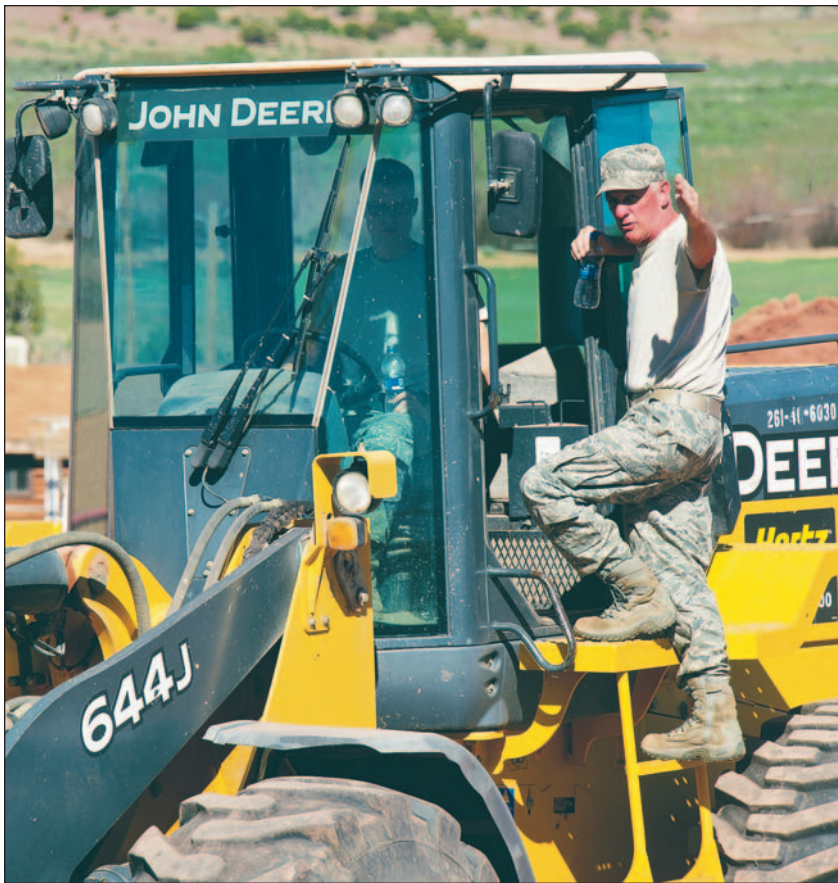
Tech. Sgt. David Cowles, right, gives instructions to Airman 1st Class Shane Kilgore during ground clearing operations at St. Michaels Association for Special Education, Window Rock, Ariz.
