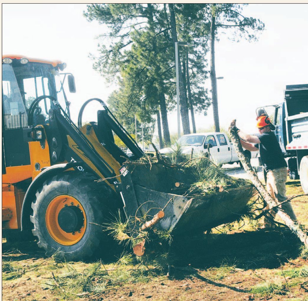
Above, 78th Civil Engineer Group workers clean up fallen branches near Bldg. 207 Tuesday.
