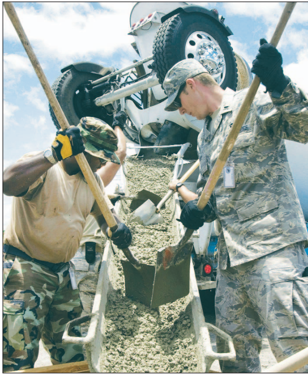
Defense Department photo by AIRMAN 1ST CLASS NICHOLAS CARZIS 1st Lt. Ryan Barry assists Staff Sgt. Brent Parker of the California Air National Guard's 146th Civil Engineering Squadron with a concrete pour in Hawaii.
