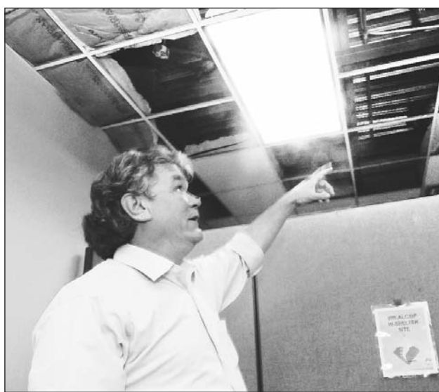
U.S. Air Force photo by SUE SAPP Mike Gavin points out where ceiling tiles and insulation are gone as a result of the water damage in Bldg. 376.
