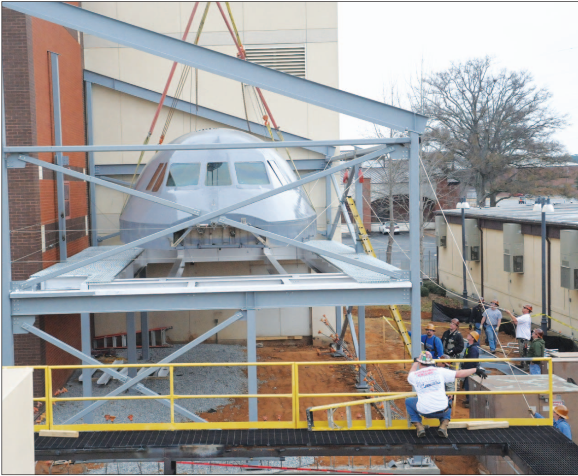
Members of the 402nd Maintenance Support Group, Industrial Services Squadron, lift the C-5 cockpit into place at Bldg. 230.
