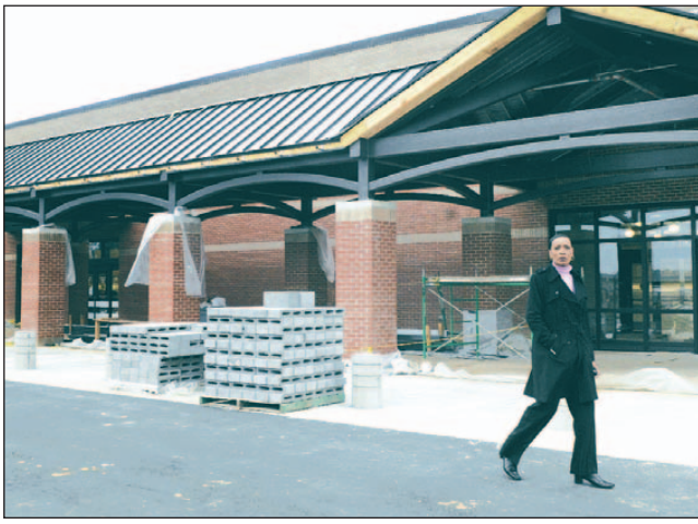
U.S. Air Force photo by SUE SAPP Paula Lewis, Defense Commissary Agency store director, said construction on the new commissary is nearly complete and the store is scheduled to open April 23.
