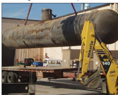
courtesy photo This 10,000 gallon propane tank buried for nearly four decades was recently raised and removed from an area near Bldg. 128. The tank became a concern last year when demolition of the building was planned.
