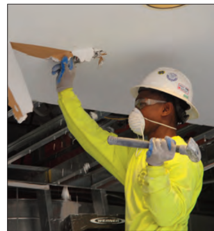
U.S. Air Force photo by RAYMOND CRAYTON Contractors are busy at work on a $29.5 million restoration and modernization project to Bldg. 700.
